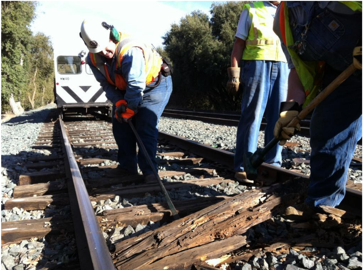
Heather uses the nipper to rip up a rotten tie
