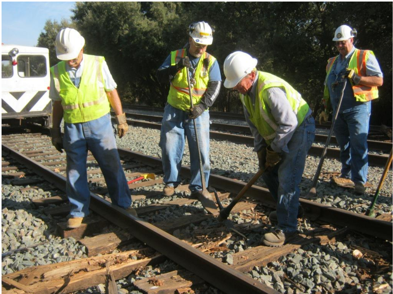
Mike T. chops away at a rotten tie while Mike F., and Chris use nippers to break-up chunks of dead tie
