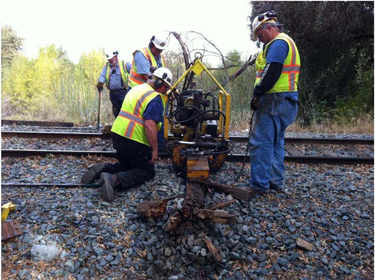
Chris, Harry, and Mike F. try to use the section-gang machine to crush – er, remove a tie
