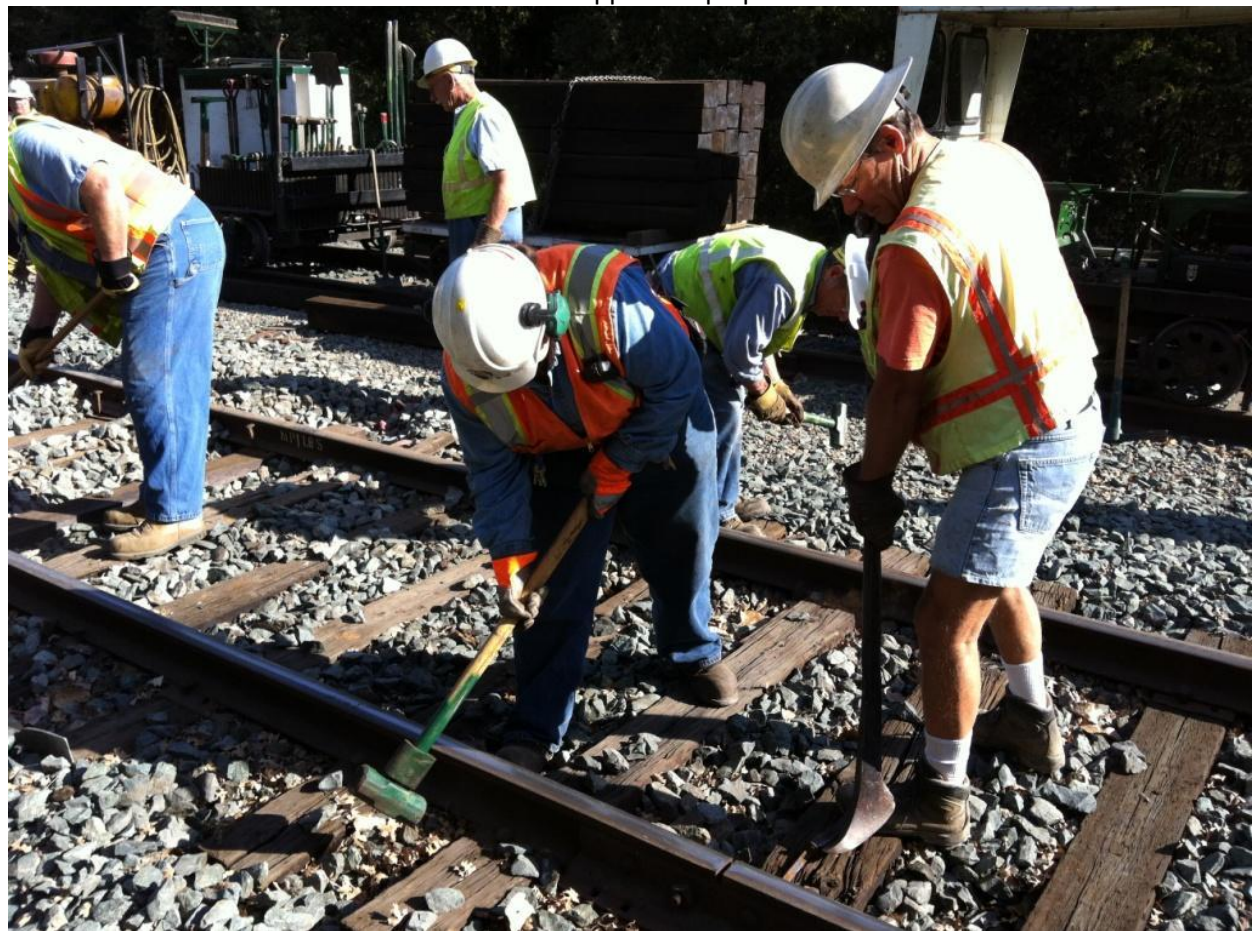
Heather and Steve work as a team at correcting a defect under a joint
